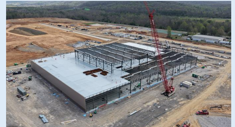
Construction and inspection activities at TRISO-X (Photos courtesy of TRISO-X, LLC)
