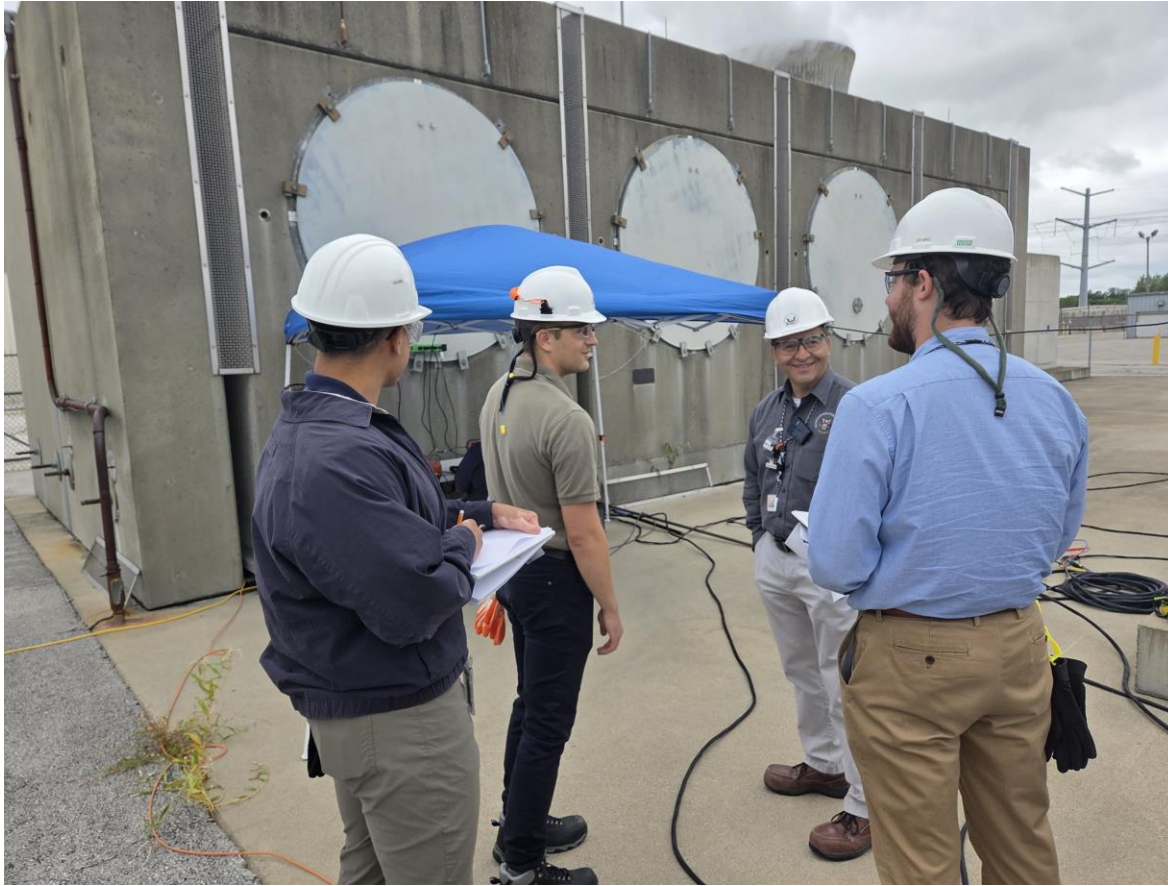
Photo: Nathan Audia, Andres Rowe, and Jake Davis inspecting at Davis-Besse, accompanied by Mohammed Shuaibi
